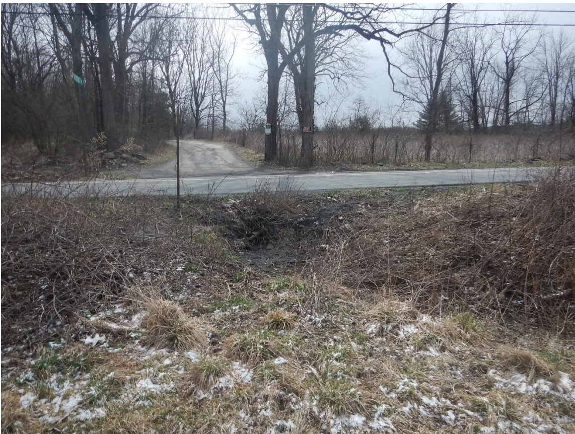
Photo 4: View of stormwater pipe, facing southeast. Photo taken 3-28-22.
