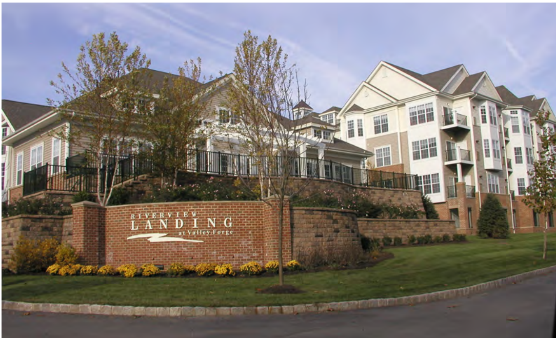
Residential development sign in West Norriton Township
