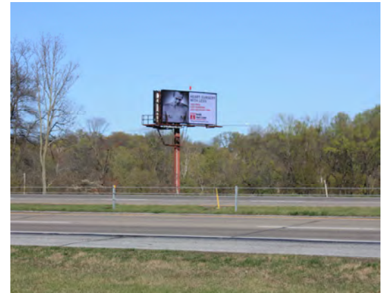
An off-premises sign located along Route 422, where the speed limit is 55 mph. A sign located along a roadway with a higher speed limit will need to be larger than those located where traffic moves slower.
