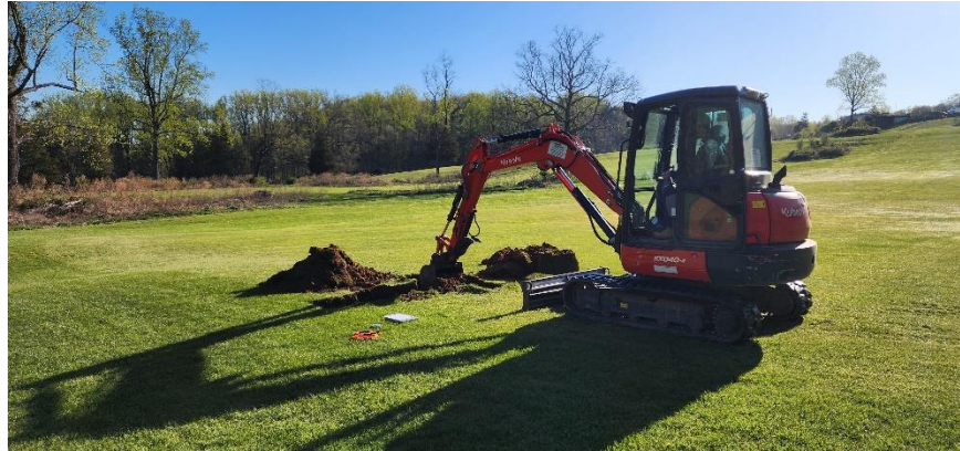
Photo #1 – TP-101 Excavation
